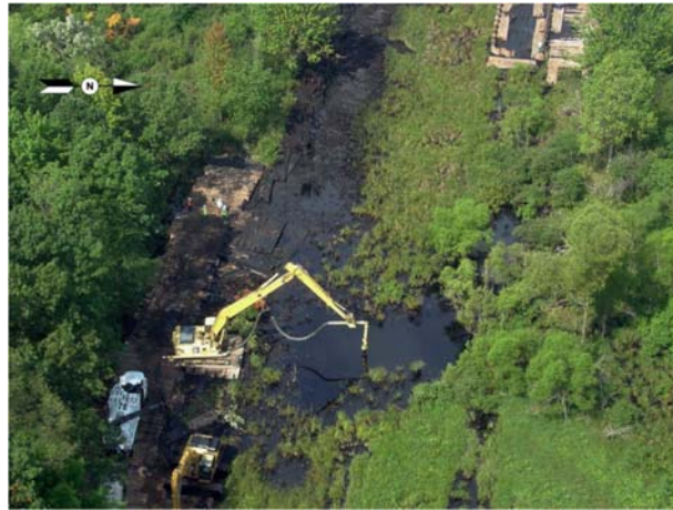
Vacuum truck on wooden matting near Line 6B spill, 2010
