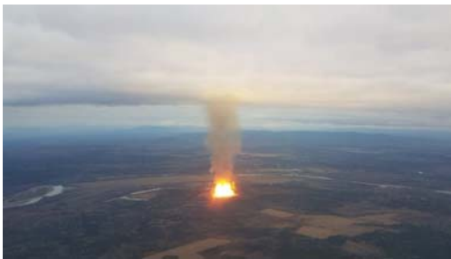
Enbridge explosion, British Columbia, 2018
